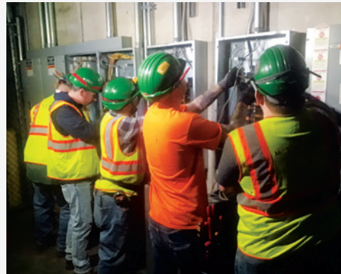
Our team working to replace (70) panelboards during the 4-hour maintenance windows.
