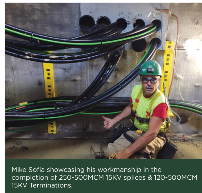
55,000 LF of conduit installed for an underground power and communications duct bank system. 110,000 LF of 15kV 500MCM power cable pulled through duct bank system. Project Foremen: Bill Peasley and Jim Gallogly
