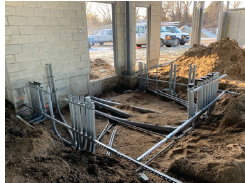
Left: Underground conduits coming into the main electrical room.
